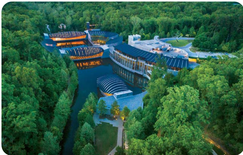
Crystal Bridges Museum's buildings and property surrounded by Ozark forests. Photo by Dero Sanford, courtesy of the Museum.
